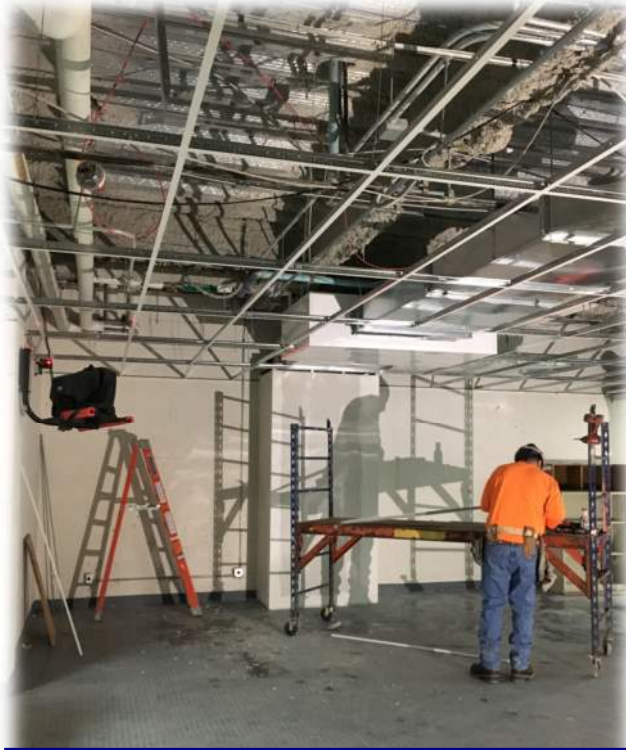
POD H Basement Ceiling Replacement
